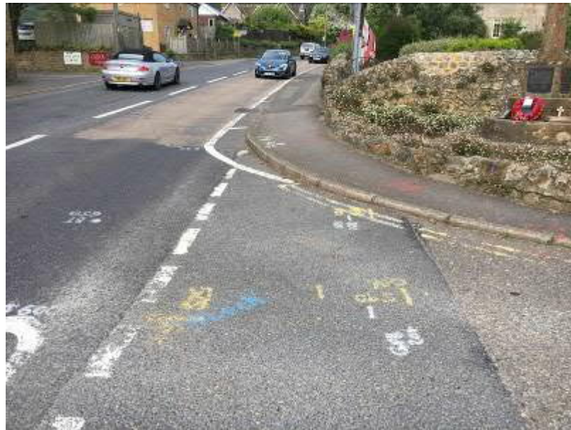
Photograph 2 – Lack of dropped kerbs on the west side of the North Road junction
