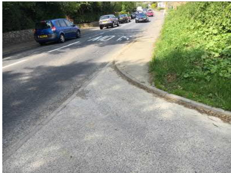
Photograph 8 – Lack of dropped kerbs at the eastern end of the northern footway
