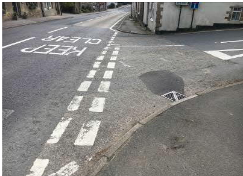
Photograph 3 – Lack of dropped kerbs on both sides of the Duck Street junction
