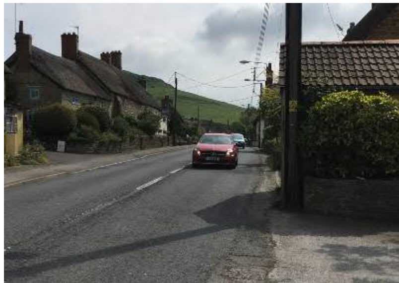
Photograph 16 – Lack of footway on the south side of the A35 carriageway
